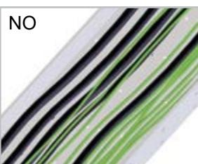
To reduce or completely eliminate the effect of electromagnetic compatibility, the basic condition is the separation of power and data cables within one tray. This can be achieved in several ways:
